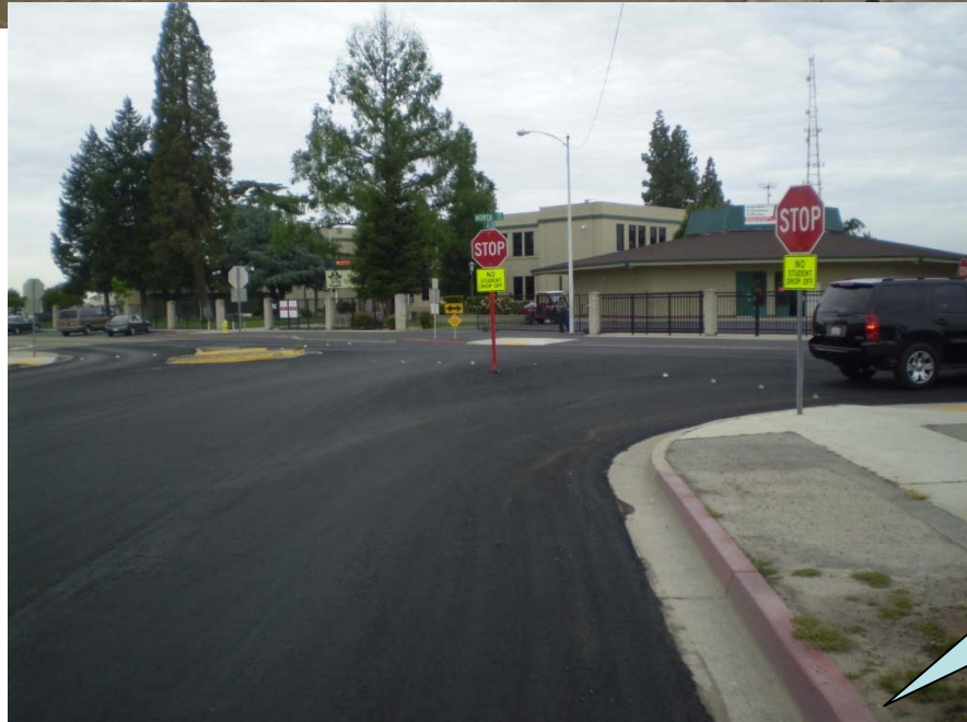
Pavement condition after 76-22TR chip seal with slurry
