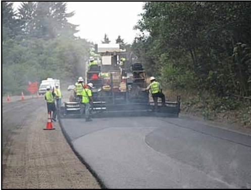
Figure 5. Behind the paver with HMA
