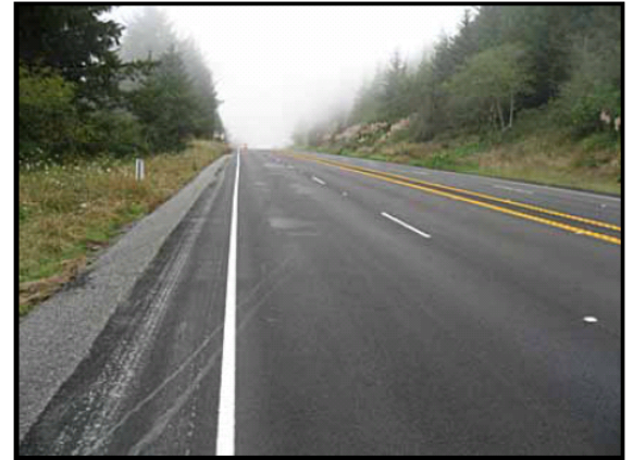
Figure 6 Finished paving with striping
