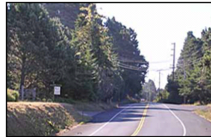
Figure 3. Finished project after striping
