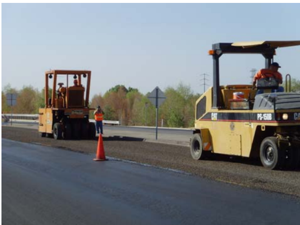
Fig. 5 followed immediately by the rollers
