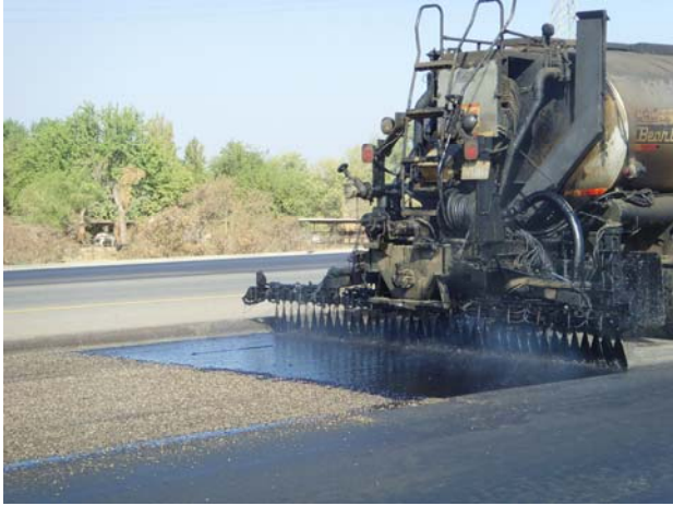
Fig. 1 spraying the asphalt binder
