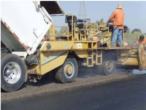
Fig. 3 laying the chip
