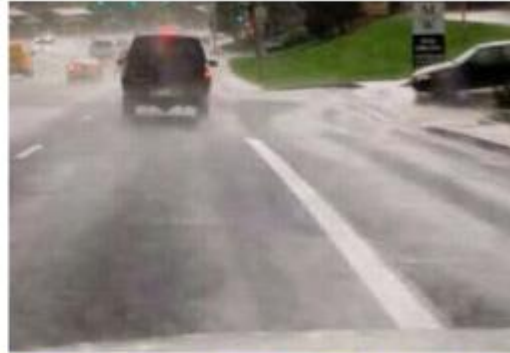
A street section paved with open-graded TBTRA shows little to no splash back, and pavement markings are clearly visible during the same storm.
