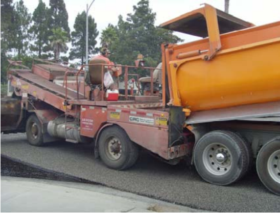
Fig. 3: laying the chip
