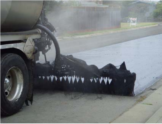
Fig. 1: spraying the asphalt binder
