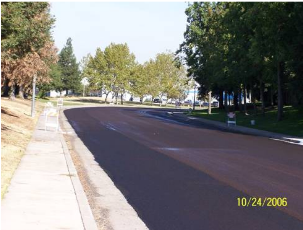
Finished Slurry Seal before fully cured
