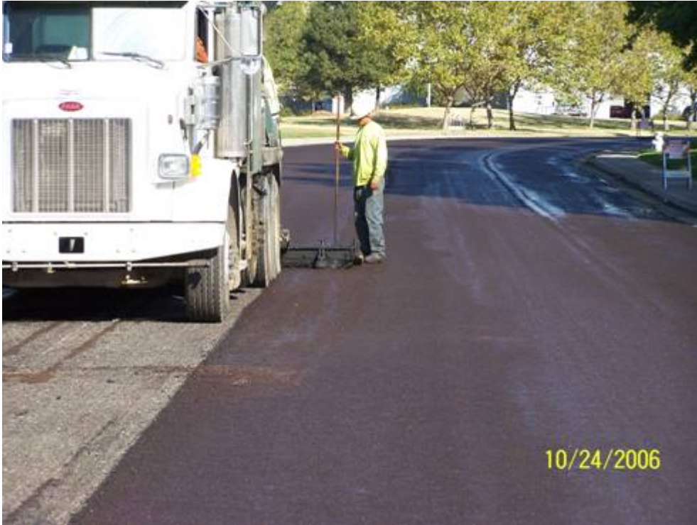
Slurry seal type 2 being placed with slurry unit
