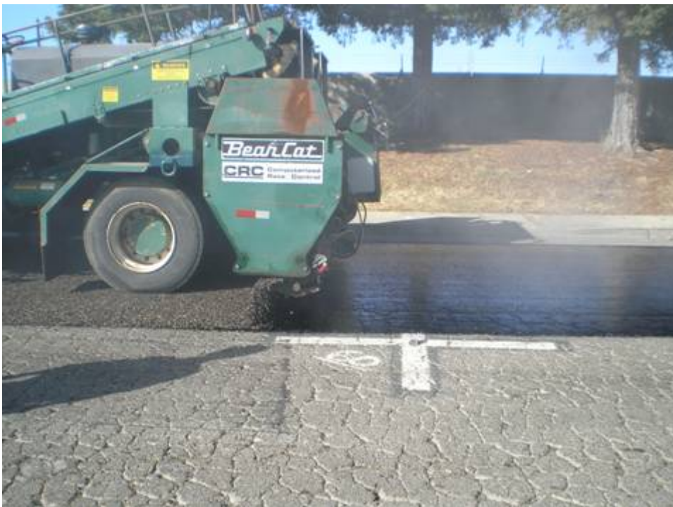
Chip spreader at work spreading product
