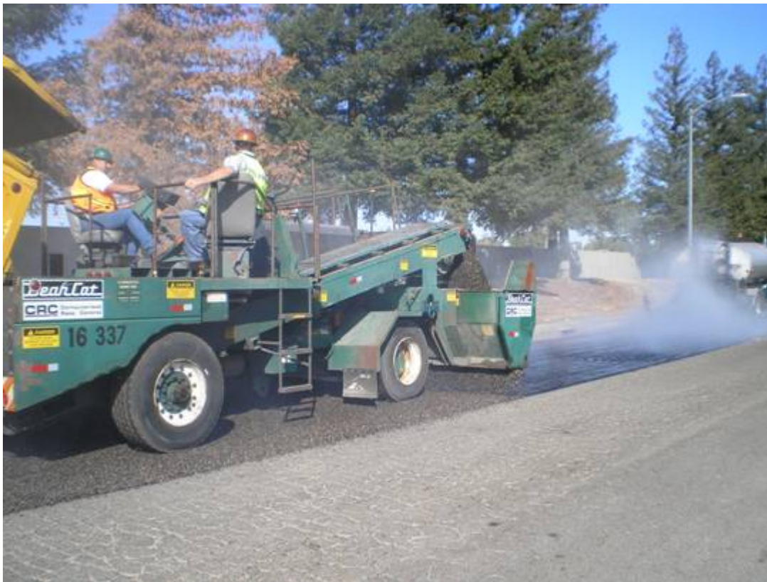
Chip spreader following distributor truck
